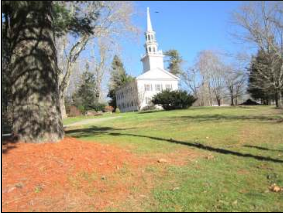
Fig. 17 Congregational Church, photo taken from Center Road facing northerly.
