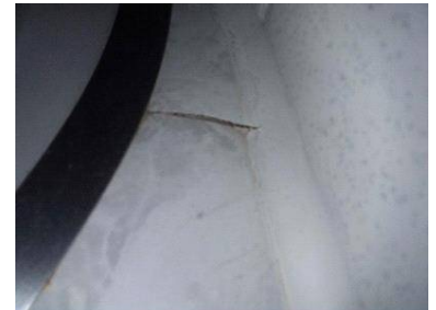
Formica is cracked and delaminating
