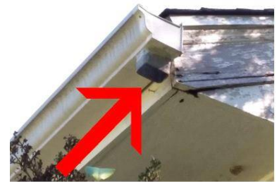
missing downspout
