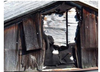
more siding damage on right side
