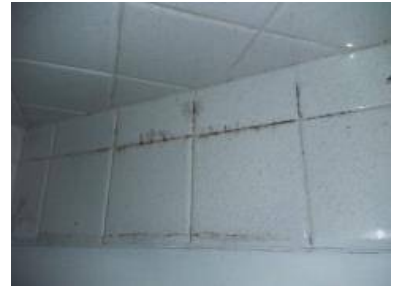
Formica is cracked and delaminating
