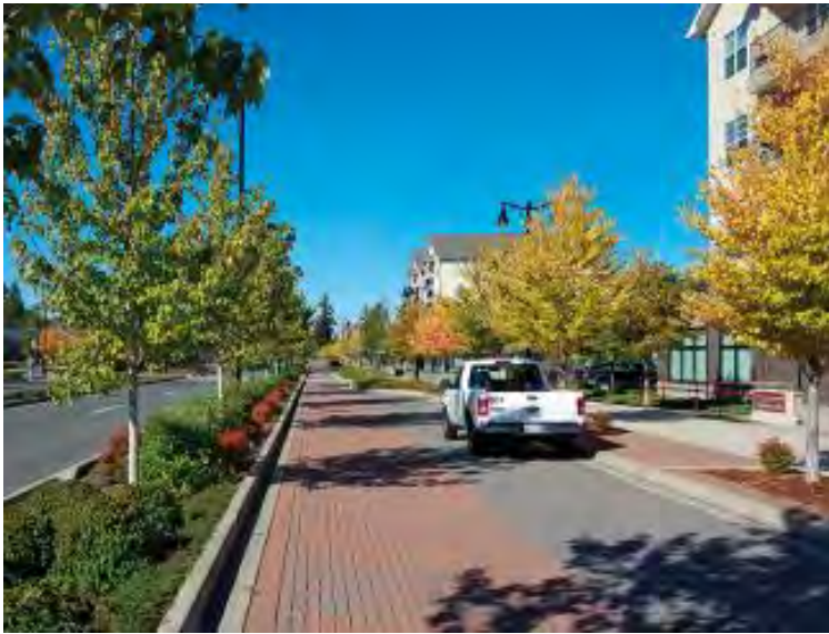
Permeable interlocking paver installation at Joint Military Base Lewis-McChord (JBLM) in Washington State. Source: https://www.estormwater.com/bmps/military-base-installs-permeable-pavers-main-street
