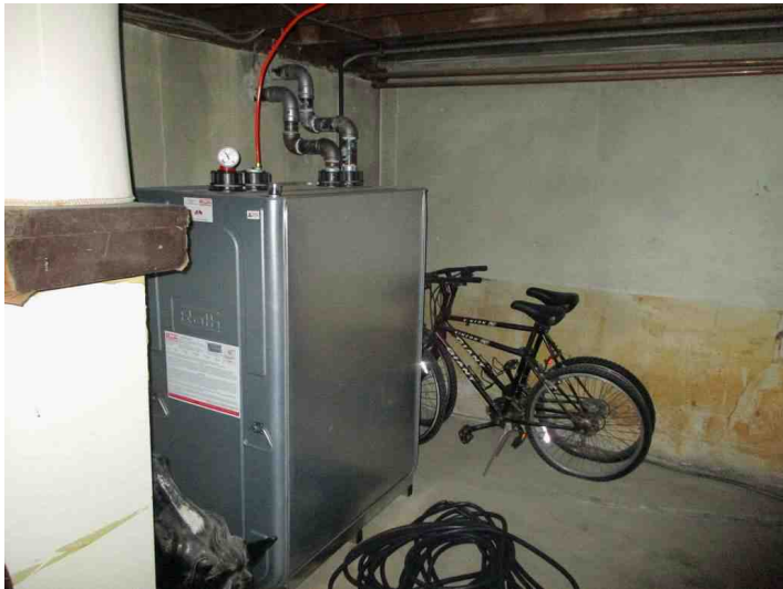
new double lined oil tank in basement
