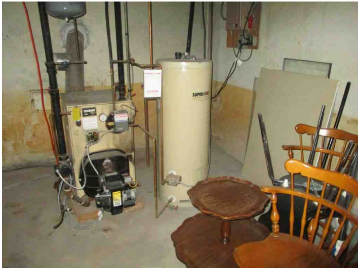
boiler & hot water heater
