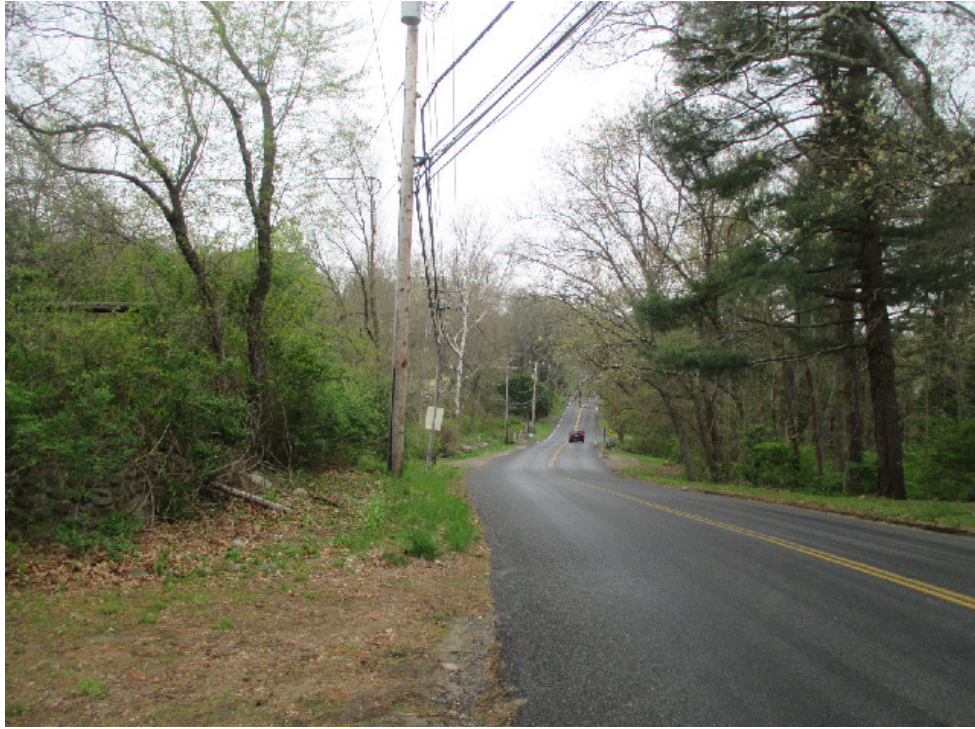
STREET VIEW - SOUTH PARK AVENUE
