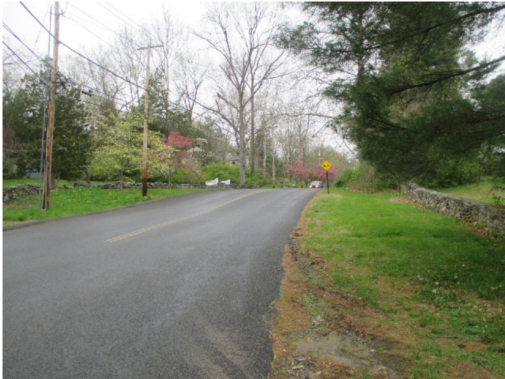
STREET VIEW - SOUTH PARK AVENUE
