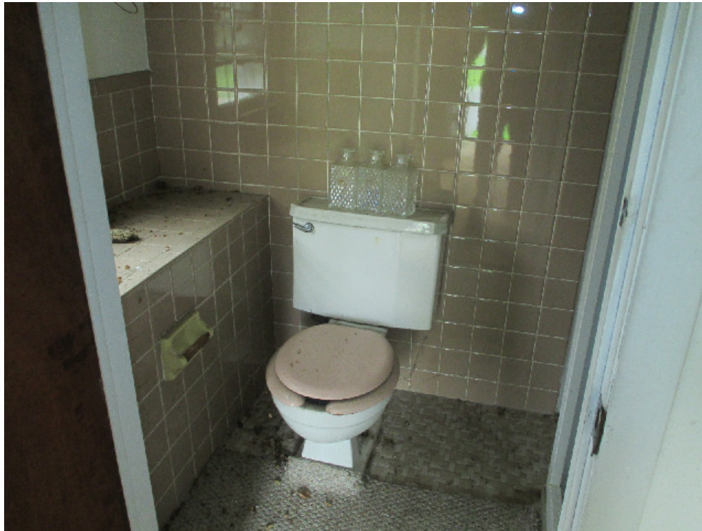
COTTAGE - UPPER LEVEL BATHROOM
